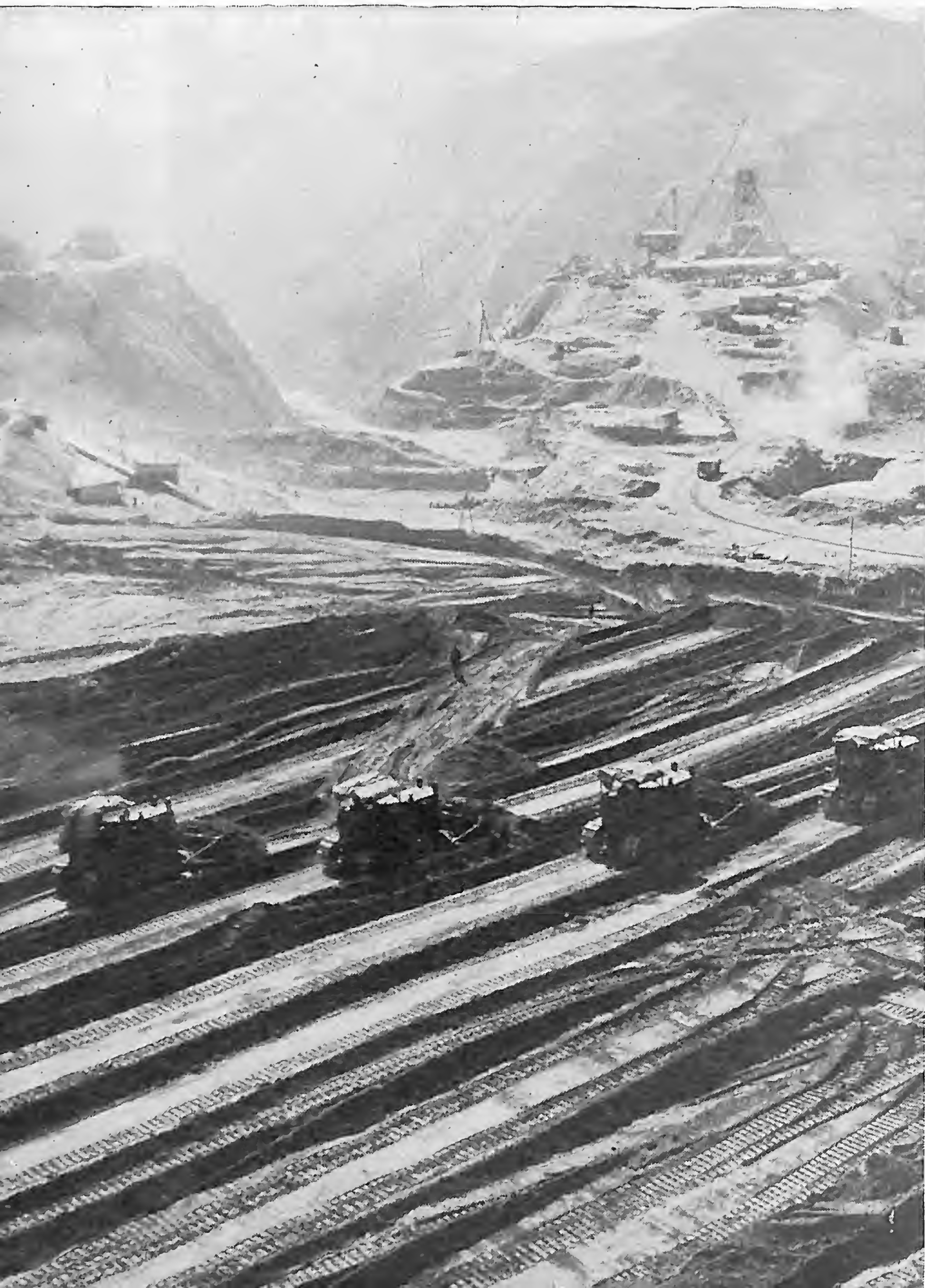
An early stage of work on the dam.
